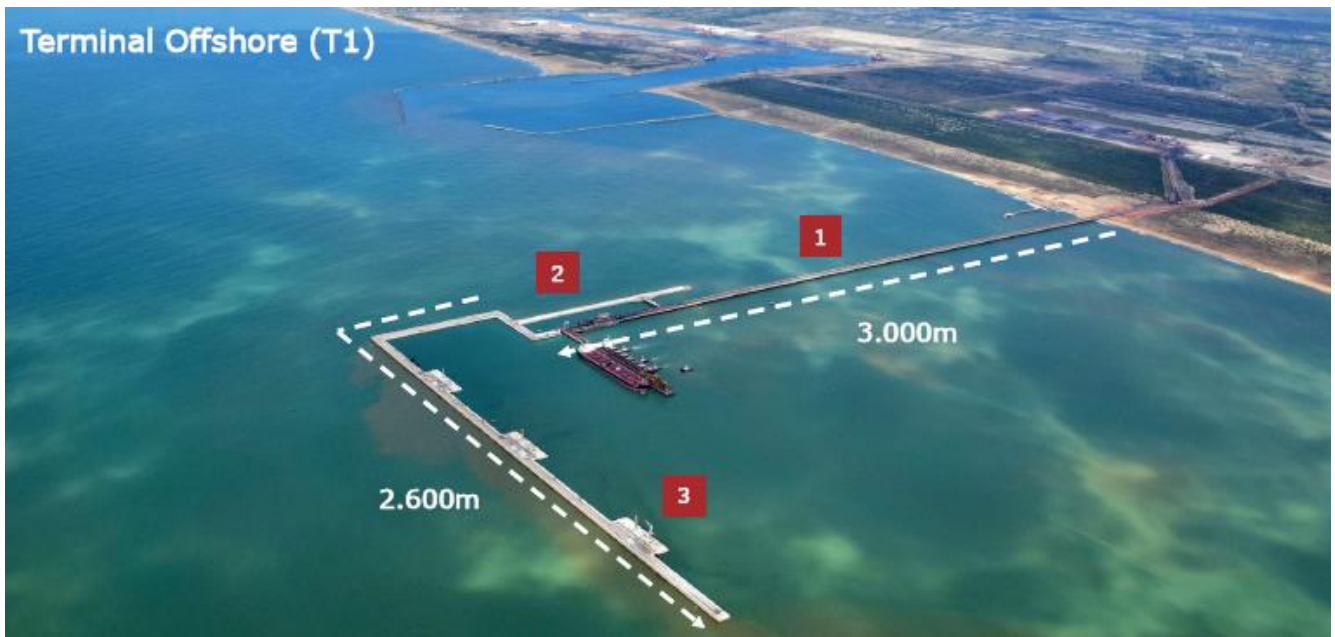
Figura 64 - Terminal Offshore T1
